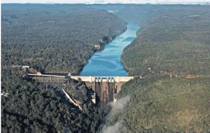
Concerns about raising the dam wall are increasing. Photos: James Brickwood
