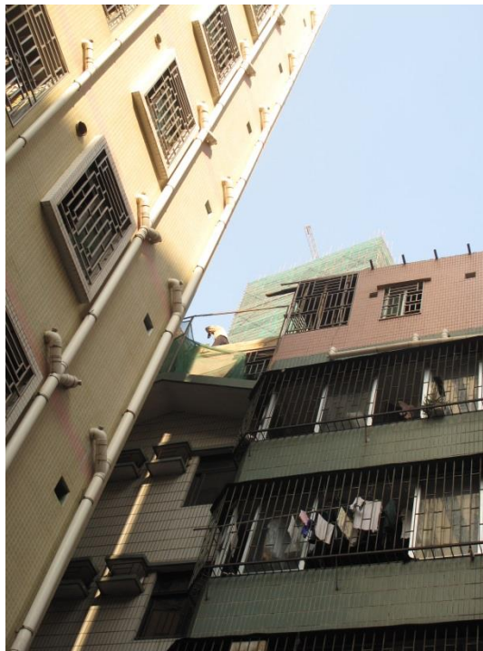
Photo 31: Qiangjian in process. Note the new living spaces being added to the existing building, all being done with the minimum safety net. Photo by author 2009
